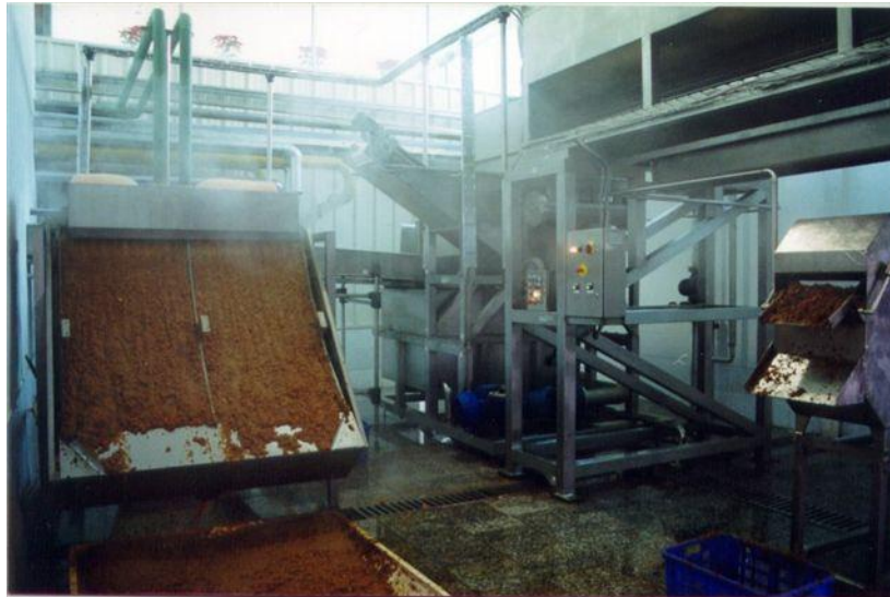
Water filtering and recovery group
