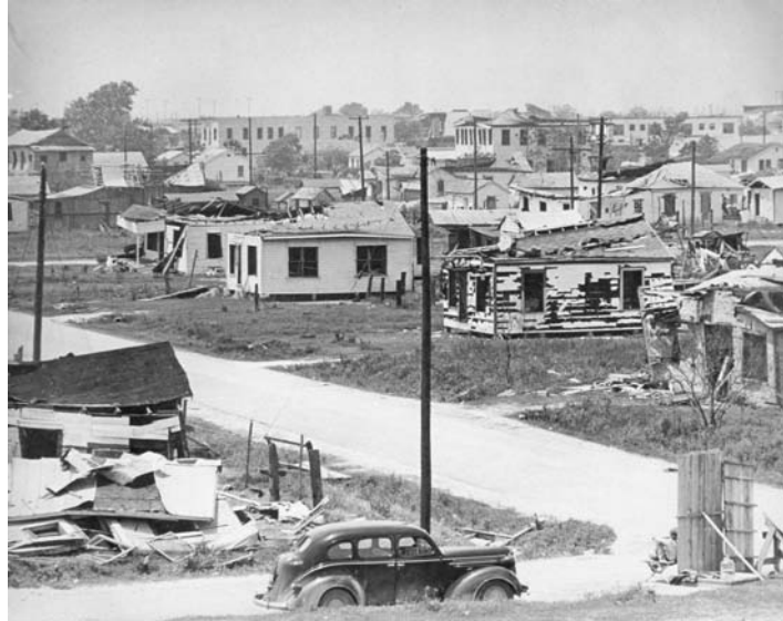
PHOTO 3: 1947 Explosion Effects in a Neighborhood
